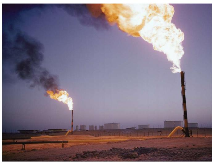
Separation or re-cycling station where natural gas that cannot be used atthe time is burned off. The tanks in the background hold crude oil that is being stored before it is sent through the pipeline to Bougie.
